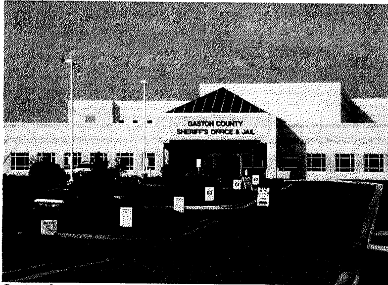
Gaston County Jail Front Elevation
