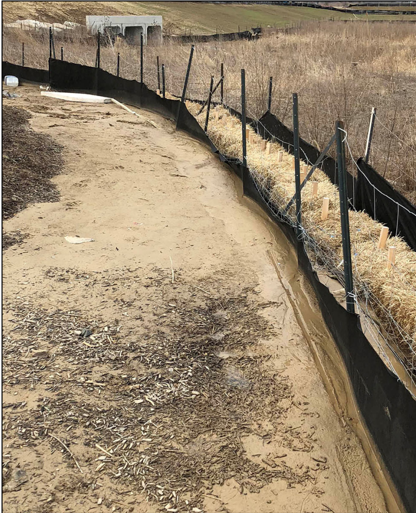
Double Row High Hazard Silt Fence (with wire backing)
